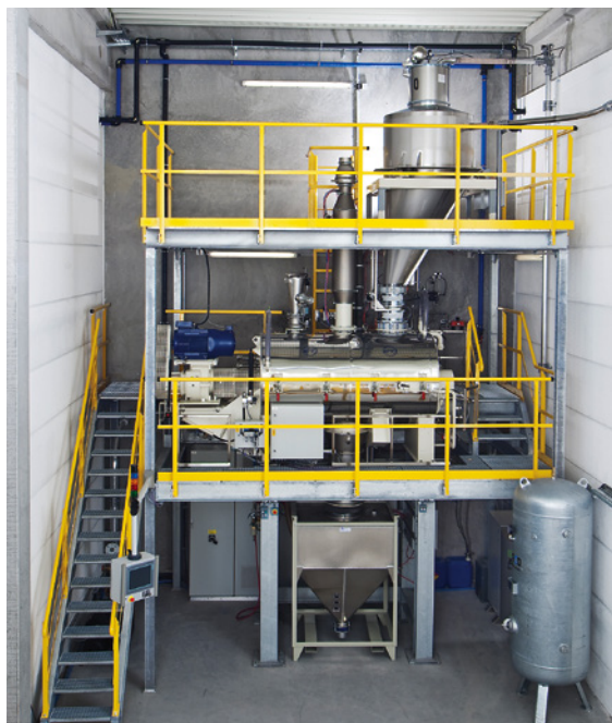
Right: A complete MTI mixing system for PE-Xa at Agru-Frank in Germany
