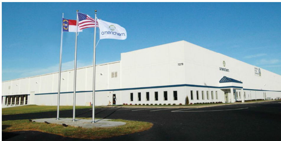
Americhem's Liberty, North Carolina plant was designed and built through the ENTEK/Americhem partnership. It employs industry-best practices to produce high quality color concentrates and compounds.
